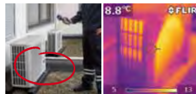
Check-up of an air conditioning installation quick and easy.
