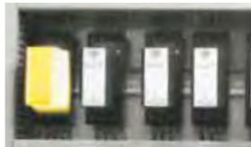
Thermal Fusion image of an overheated circuit breaker
